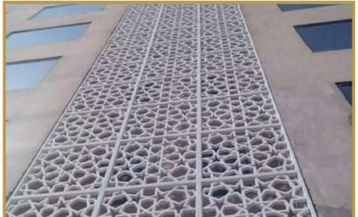
Duct Pipe Covers
